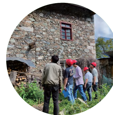
Assessing earthquake-damaged buildings and conducting urgent evaluations.
